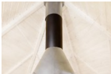
Grill Chimney Extension
